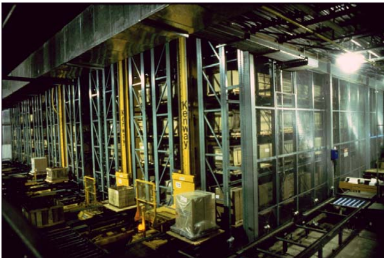
Figure 16.2. Unit Load Automated Storage/Retrieval System
