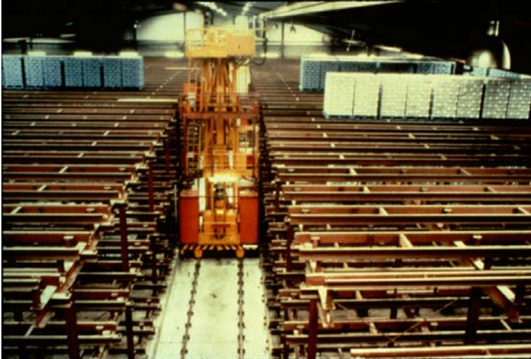
Figure 16.48. Deep Lane Storage System Example
